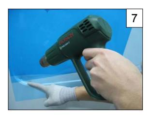
Heat the material up to 45-55°C and stretch the material in the corrugation:
